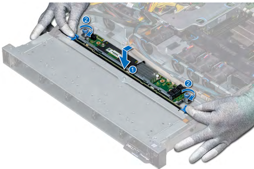
Figure 72. Installing the hard drive backplane
