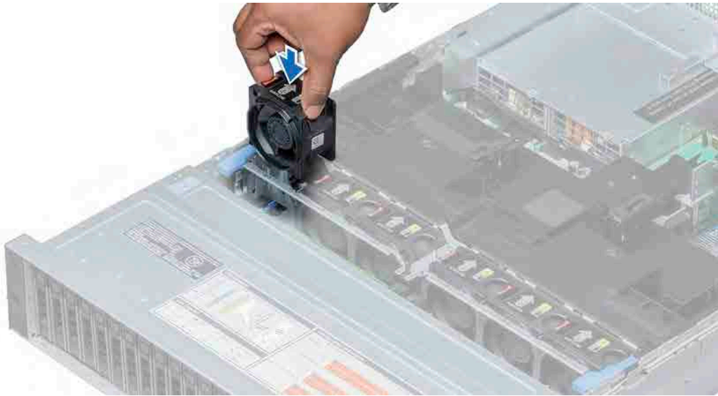
Figure 30. Installing cooling fan
